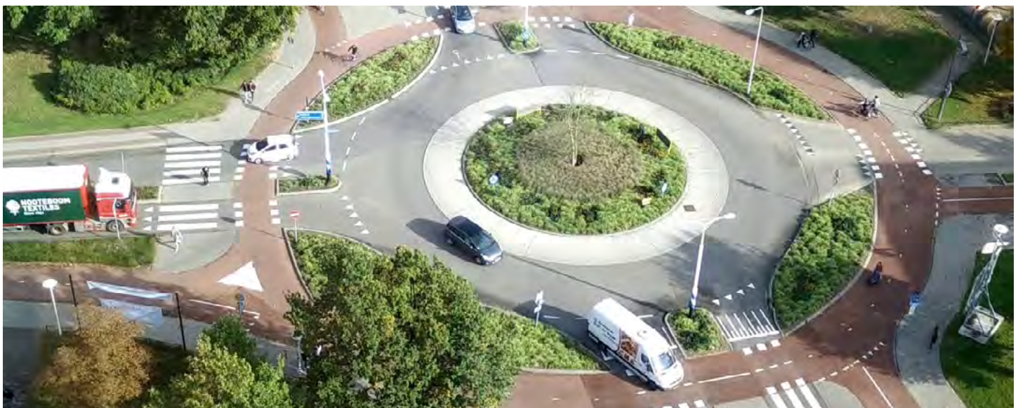
Exhibit 2.34: Dutch roundabout with bi-directional cycling lanes | Source: Frank van Caspel
