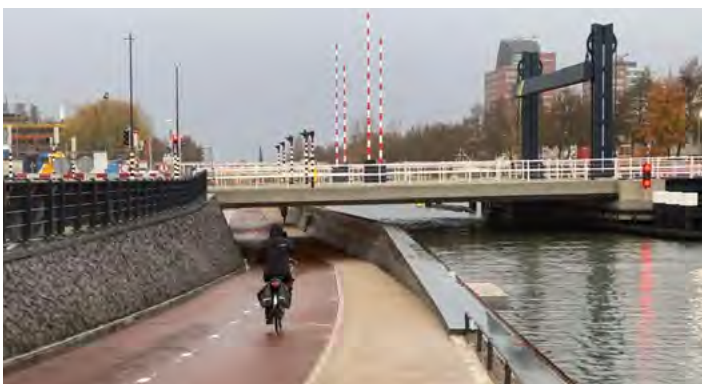
Exhibit 4.12: Bike underpass in Utrecht | Source: Bicycle Dutch
