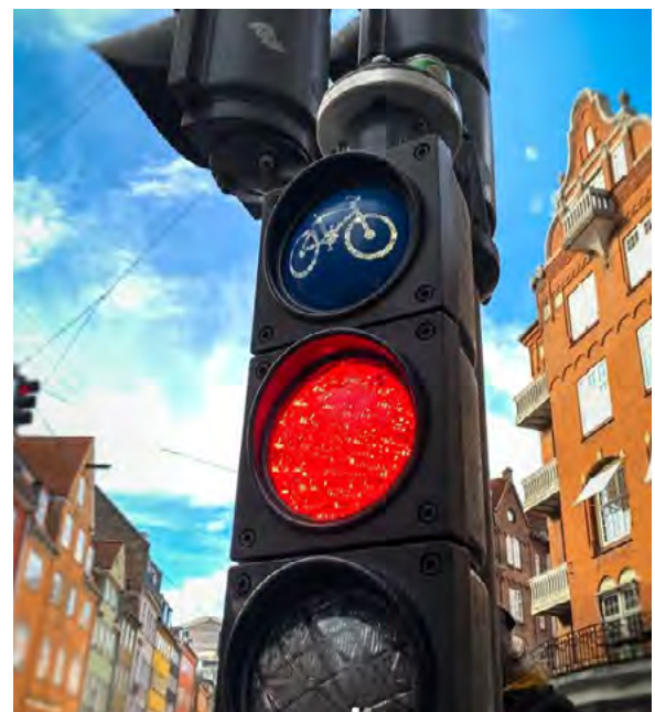
Exhibit 8.5: Rain sensor on traffic signal Source: @Denmarkdotdk
